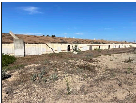
Typical Building Exterior - All Buildings
