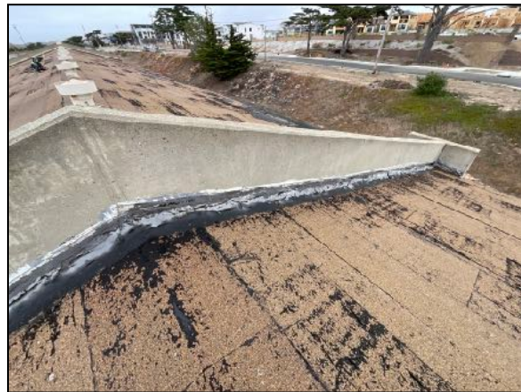
Typical Roofing - All Buildings
