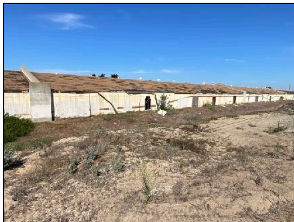
Typical Building Exterior - All Buildings
