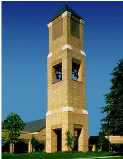
A bell tower
