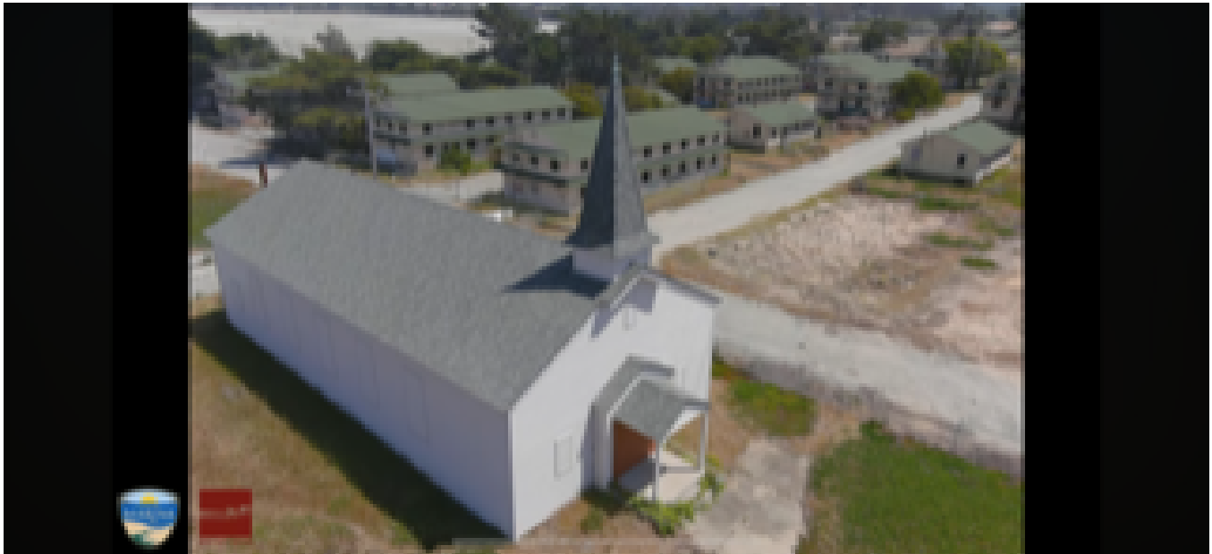
PRE-CONSTRUCTION PHOTOS: DUNES CITY PARK
