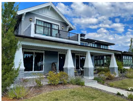
Balcony and covered front porch entry.
