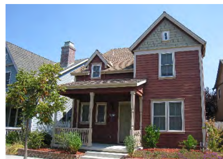
Porch entry provides weather protection.
