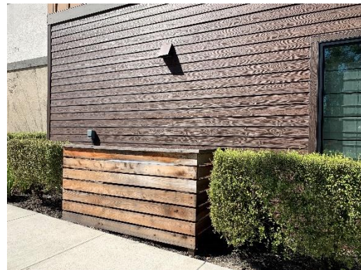
Screened mechanical equipment and vents painted the same color as the adjacent building façade.
