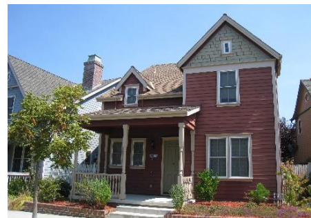
Porch entry provides weather protection.
