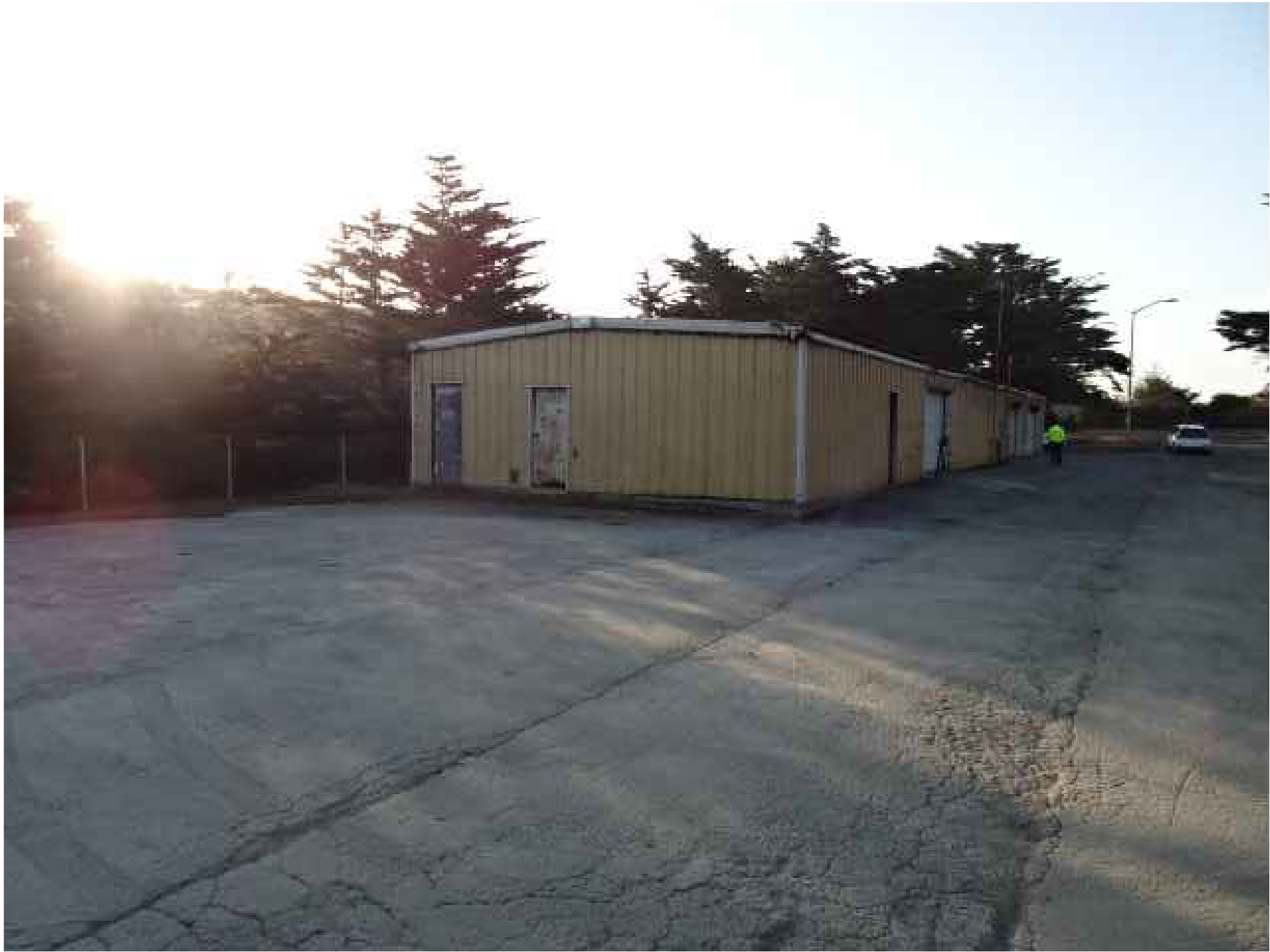
SOUTHEAST VIEW OF METAL BUILDING
