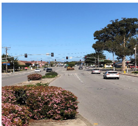
Figure 2-8. Reservation Road functions as an arterial street.
