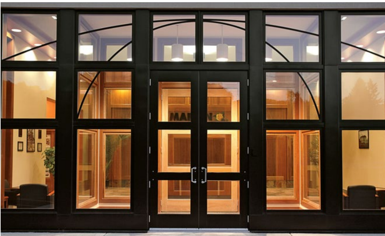
Building entry with transom window.
