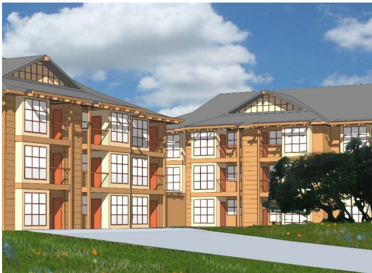
Junsay Oaks Apartments.
