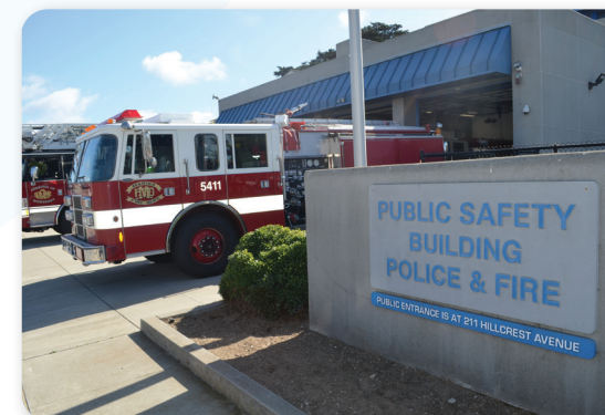
Marina's public safety facilities were built to protect a much smaller city, resulting in slower emergency response times.
