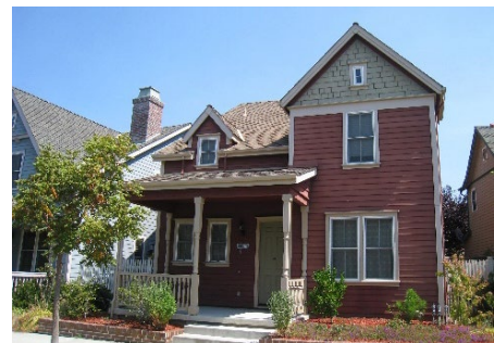
Porch entry provides weather protection.
