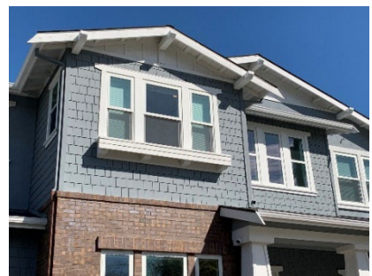
Decorative eave detailing, window lintels, and window boxes.
