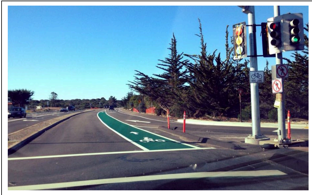
Figure 3.1-4: Imjin Parkway Bike Lane with Green Paint
