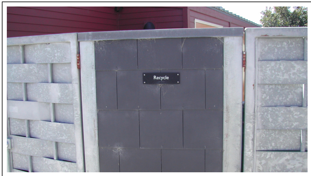
Figure 2.4-9: Designated Recycling Enclosure
