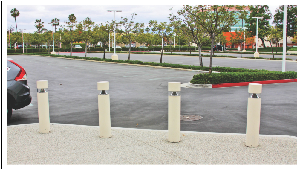
Figure 2.5-16: Pedestrian Scale Bollard Lighting
