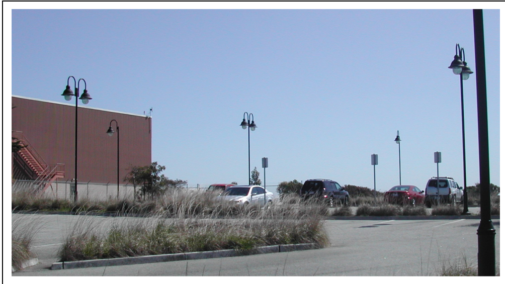
Figure 2.4-10: Parking Lot Lighting
